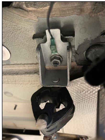
Figure 31: Ground Prep and Install
